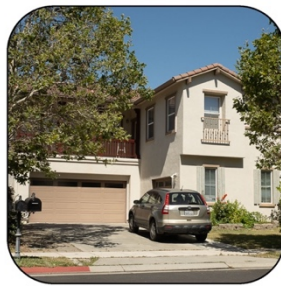
Parking garage/carport in front
