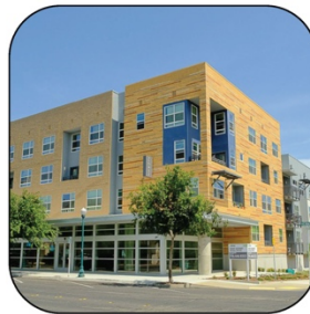
Set forward with continuous but separate façade
