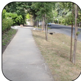
Sidewalk with trees, landscaping, and drainage swale (no curb)
