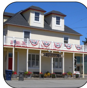
Shops face street with housing above
