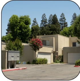
Stepped back and façade with many parts
