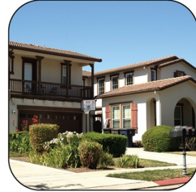
Garage setback, landscaped yard
